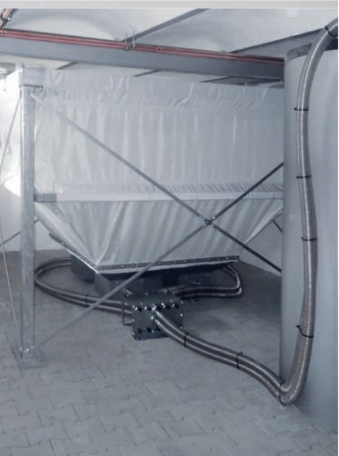
Flexilo MODULE with 4 discharge units in a boiler room
